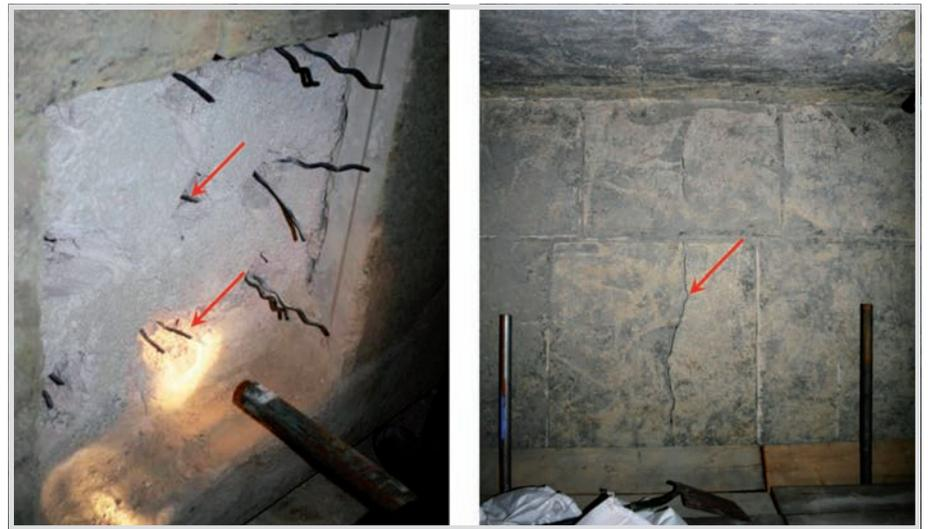
Fig. 9. Anchor ruptures and separation cracks in refractory concrete as a result of hindered slab curvature.
